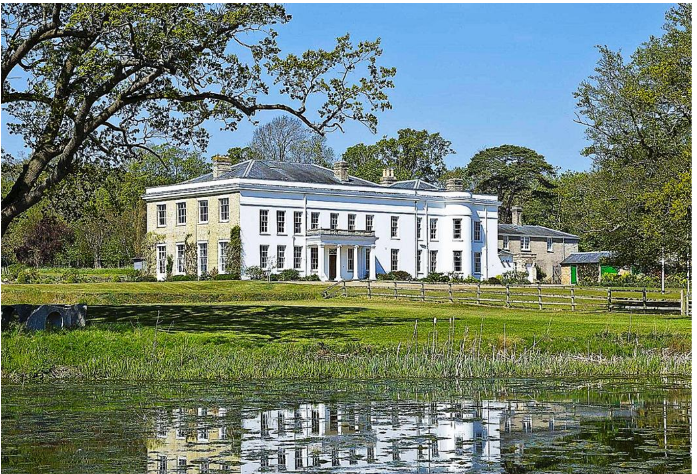
The façade of Little Haugh Hall.
