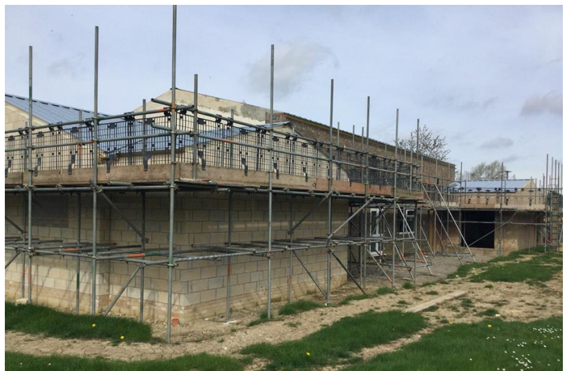
These photographs hardly show it, but the roof is on.
